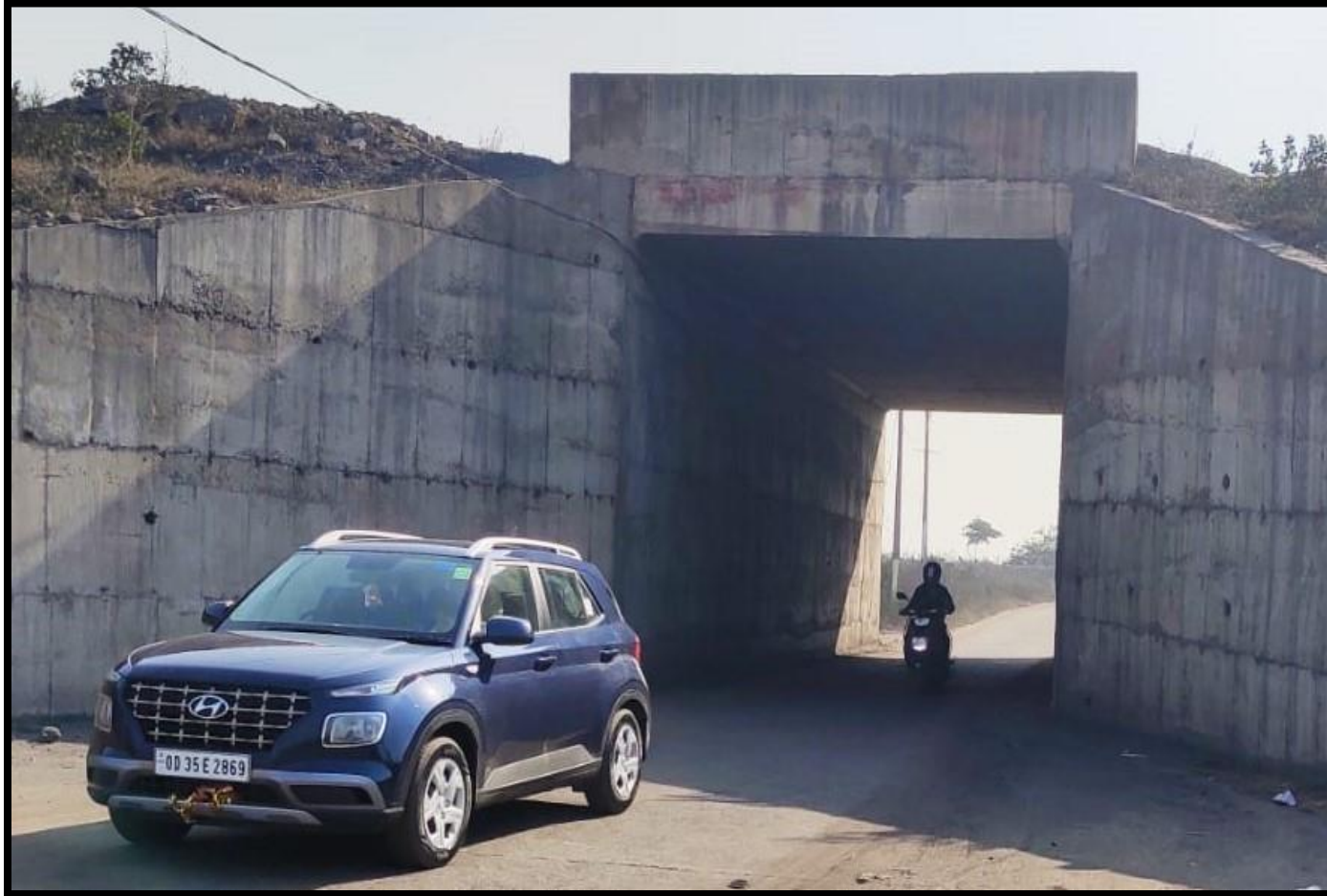
SISHU MANDIR CHOWK-UNDERPASS
