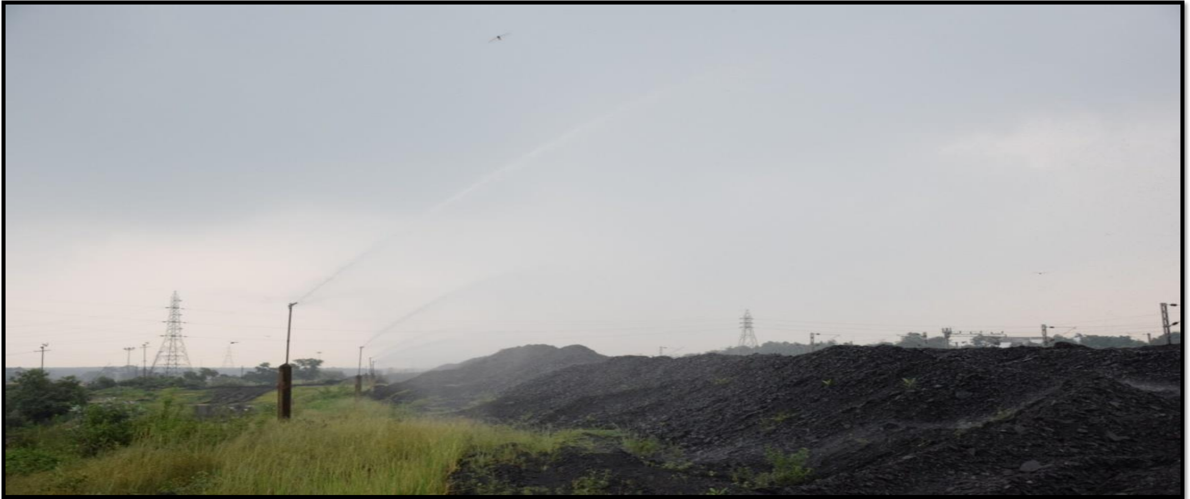
Fixed sprinklers in operation at siding no. 1 & 2
