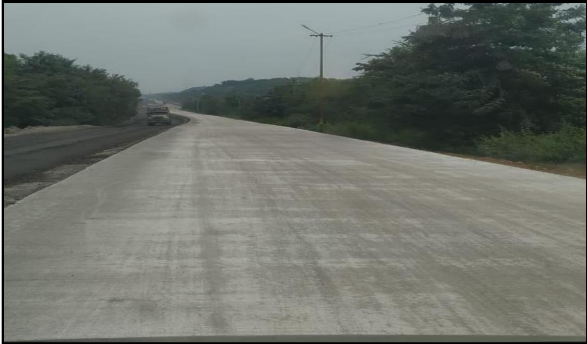
CONCRETE COAL TRANSPORTATION ROAD CONSTRUCTED AT BHUBANESWARI OCP
